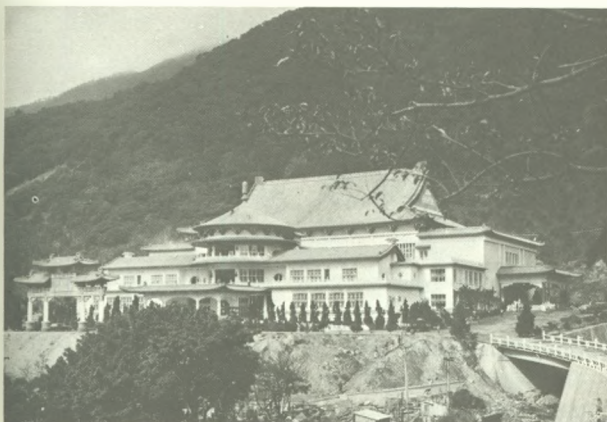
DEDICATED in November by General Chiang Kai-shek, the Chungshan building near Taipei is the most recent undertaking in memory of the late Chinese political leader, Sun Yat-sen.
