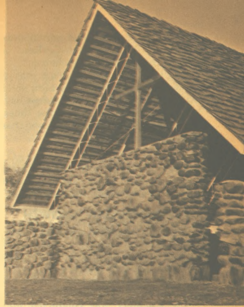
AN OPEN AIR stone chapel, built adjacent to the hospital complex.
