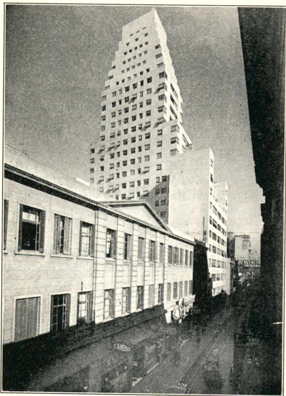
29-story "Safico" building, Buenos Aires, Argentina.
